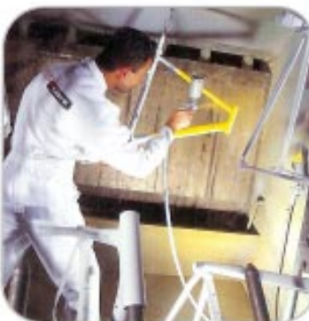
Application manuelle de la peinture. Hand spraying.
